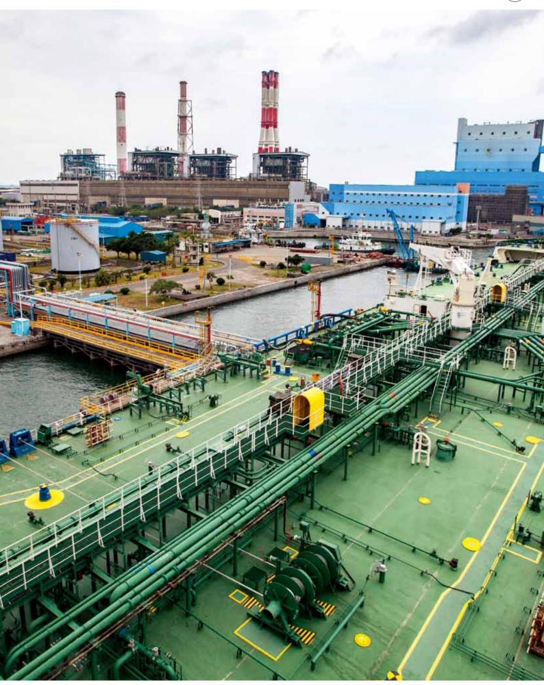
The Dalin Refinery was originally established as a part of the Kaohsiung complex but in 1996 was hived off as an independent operation. Its daily capacity is 300,000 barrels, with both incoming crude and outgoing refined products handled by four offshore mooring and unloading buoys and dedicated port facilities.
