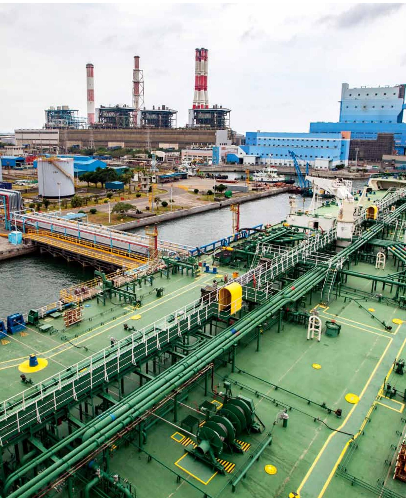
The Dalin Refinery was originally established as a part of the Kaohsiung complex but in 1996 was hived off as an independent operation. Its daily capacity is 300,000 barrels, with both incoming crude and outgoing refined products handled by four offshore mooring and unloading buoys and dedicated port facilities.
