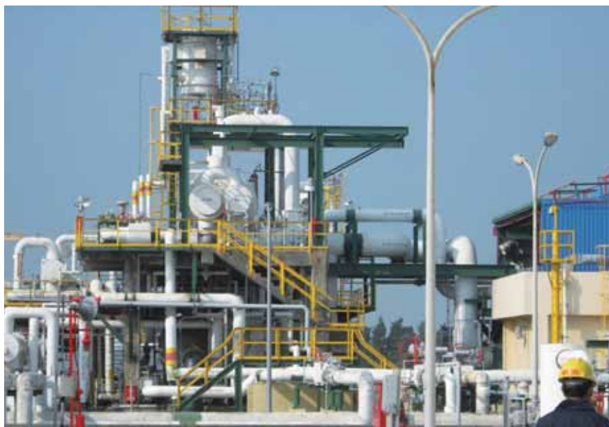
Cold energy power generation cycle system at Yongan LNG Plant
