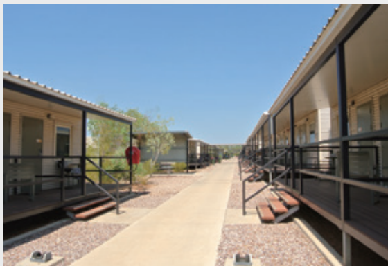
▲ Minigurr-Ma Accommodation Village 員工宿舍外觀。
