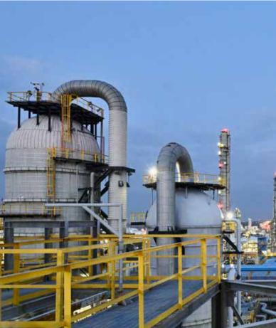
a 144,000-ton-per-year methyl tert-butyl ether (MTBE) unit, together with associated technology, in order to boost the added-value of the mixed C4 hydrocarbons produced by the RFCC unit. The project was fully commissioned when volume production began in 2016.
