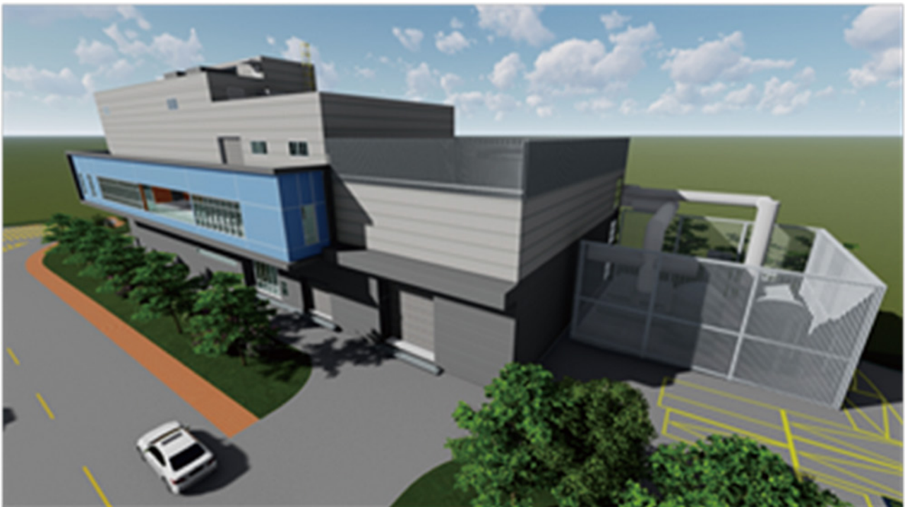
Vision of the new construction of safety testing laboratory of battery electrical energy storage (Hsinchu Science and Technology Park - Tongluo campus Testing service is scheduled to be available in January 2025)
