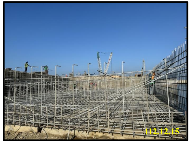
B22 堤面鋼筋綁紮
