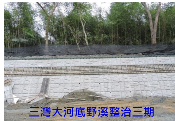
(C) 護岸開挖後方草叢設置黑紗網
