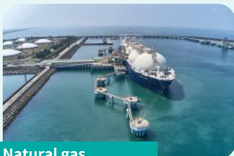
Natural gas receiving station
