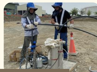
Groundwater circulation well method
