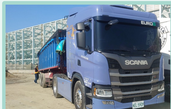
Transportation of soil away from Kaohsiung Refinery
