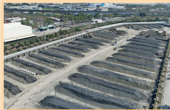
Bioremediation supplies for section 3 of Kaohsiung Refinery, temporarily stored at section 6-3
