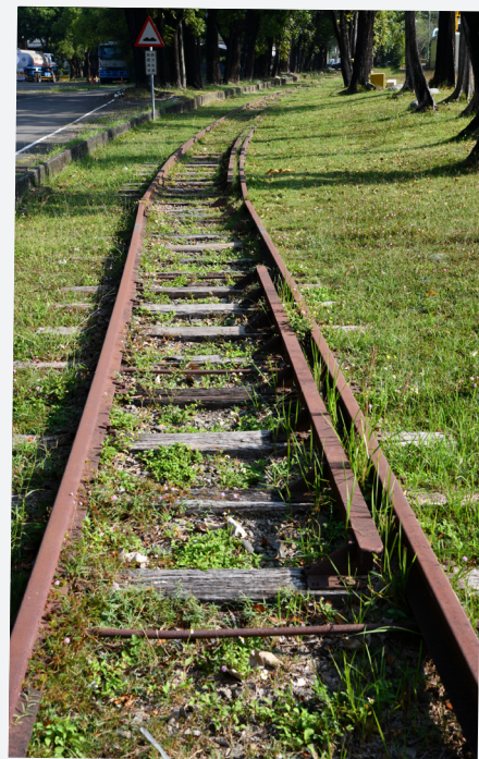
Tank truck rails
