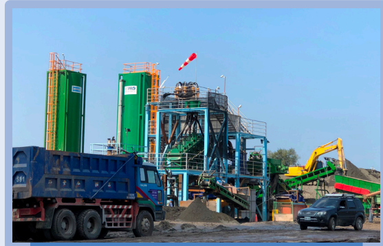
Asia New Bay Area - soil washing equipment at Temao Ernan Site
