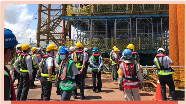
Contractor management - on-site audit
