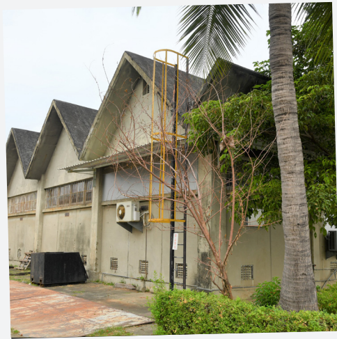
Warehouse of the 6th Fuel Plant
