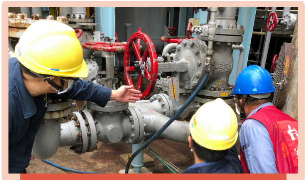
Contractor management - pre-work inspection
