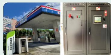
Hualien Guangfu Station: verify mobile LTO energy storage system
