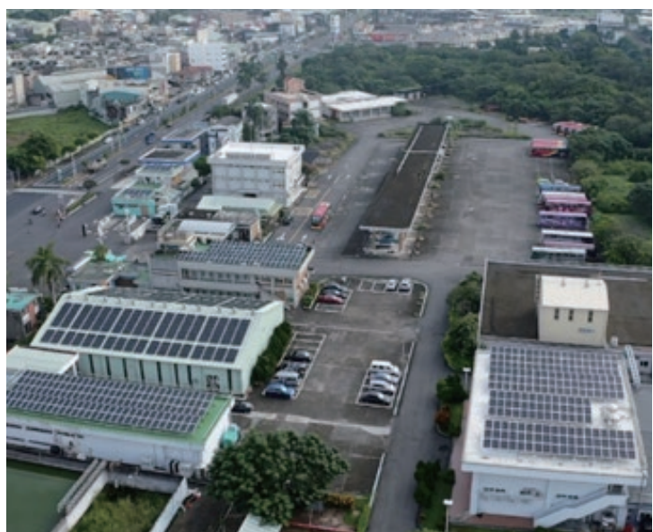
PV system at Chiayi Technology Park
