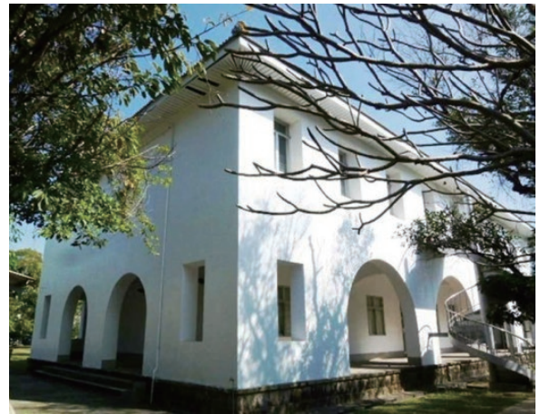
Main office corridor and arched doors
