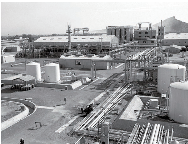
The First Naphtha Cracking Facility at Kaohsiung
