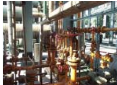
將軸封閘閥更換 BELLOWS SEAL TYPE 減少軸封逸散
